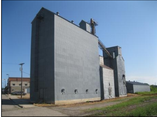
M & St. L Elevator, original 1886 elevator located in the middle (2012)
